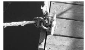
On the left is a great way to place permanent dock lines. The cleat is still relatively free for visitors to use.
