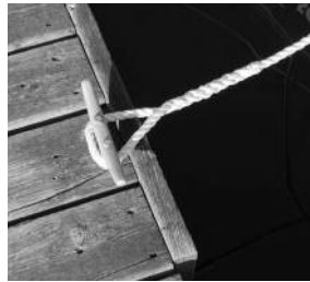
Above: a proper splice fitted well to the cleat.
